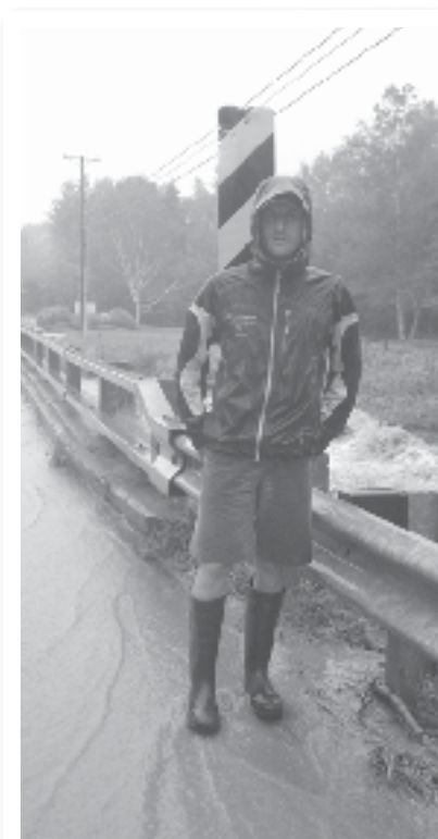
Jamie Belchak, Rehab Manager, checking out flooding in Killington
